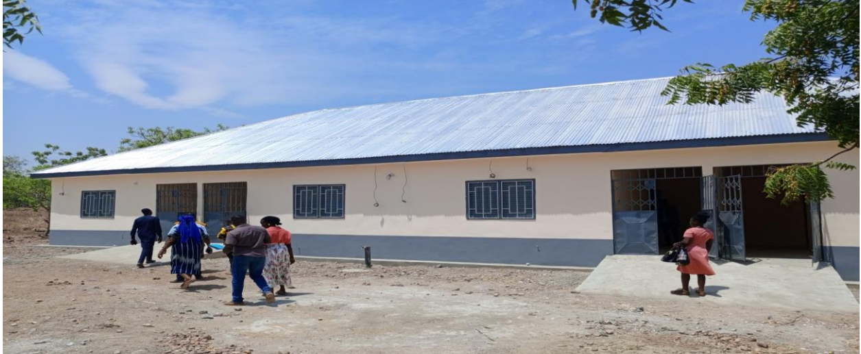
Constructed Nurses bangulow at Nangodi- DACF RFG
