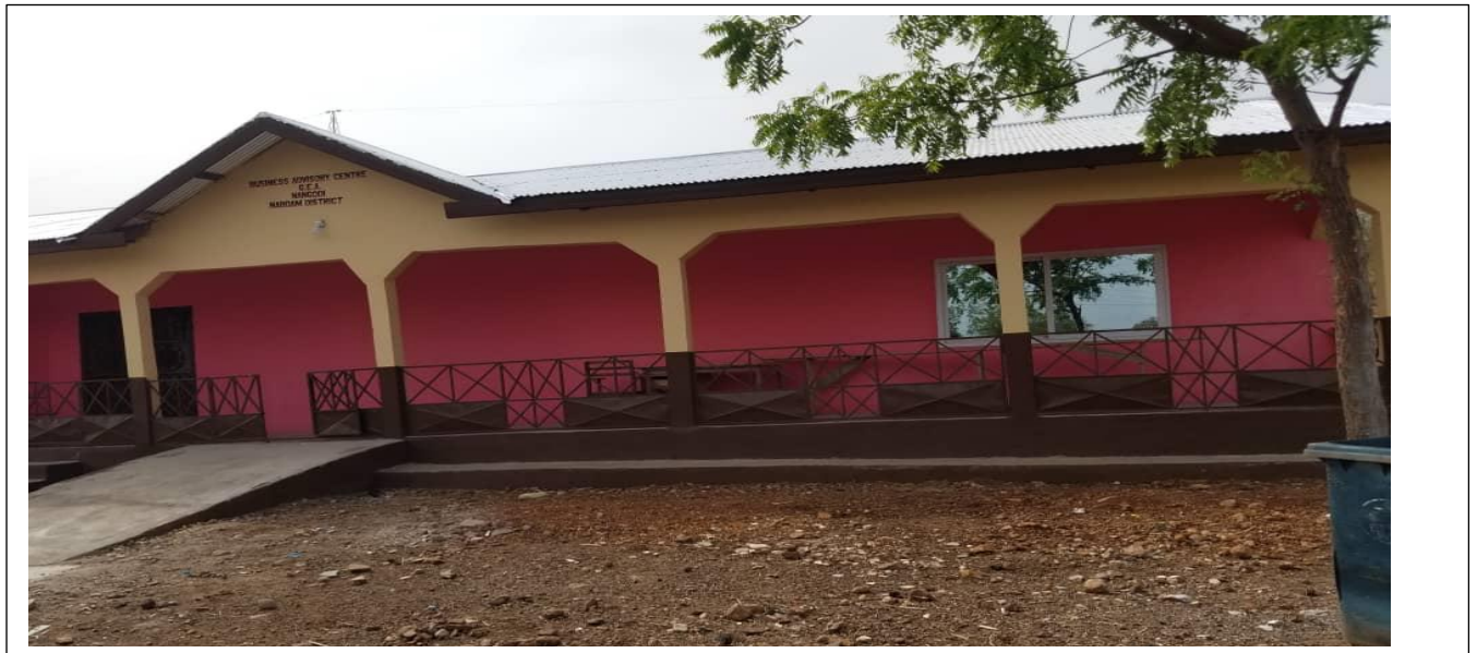
Completed the construction of Business Adversary Centre District Office
