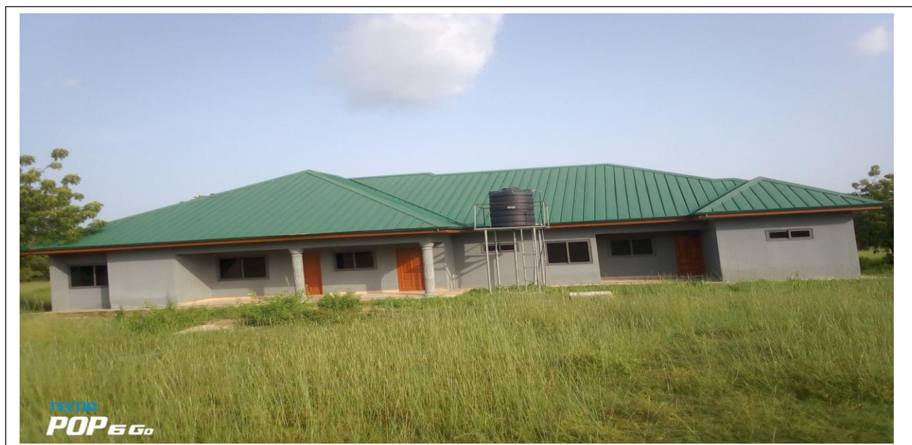
DCE Bungalow constructed-DACF-RFG
