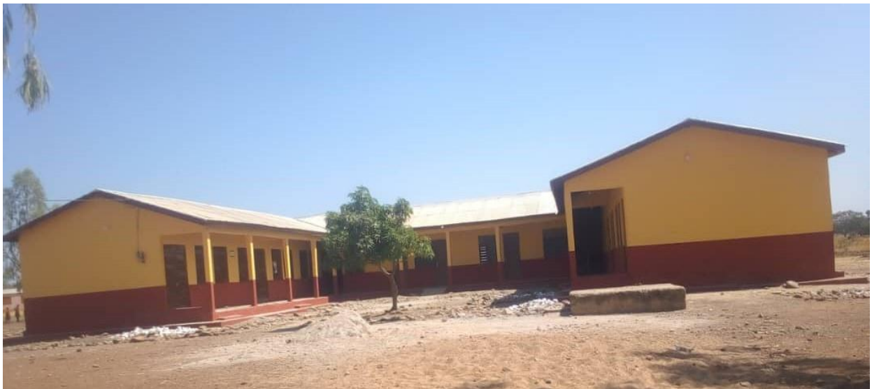
Rehabilitated 6-unit classroom block at Dagliga-SOCO
